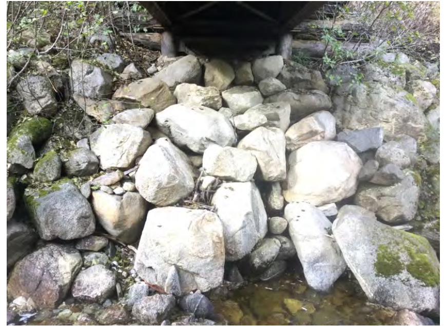
Left Bank Abutment when facing downstream
