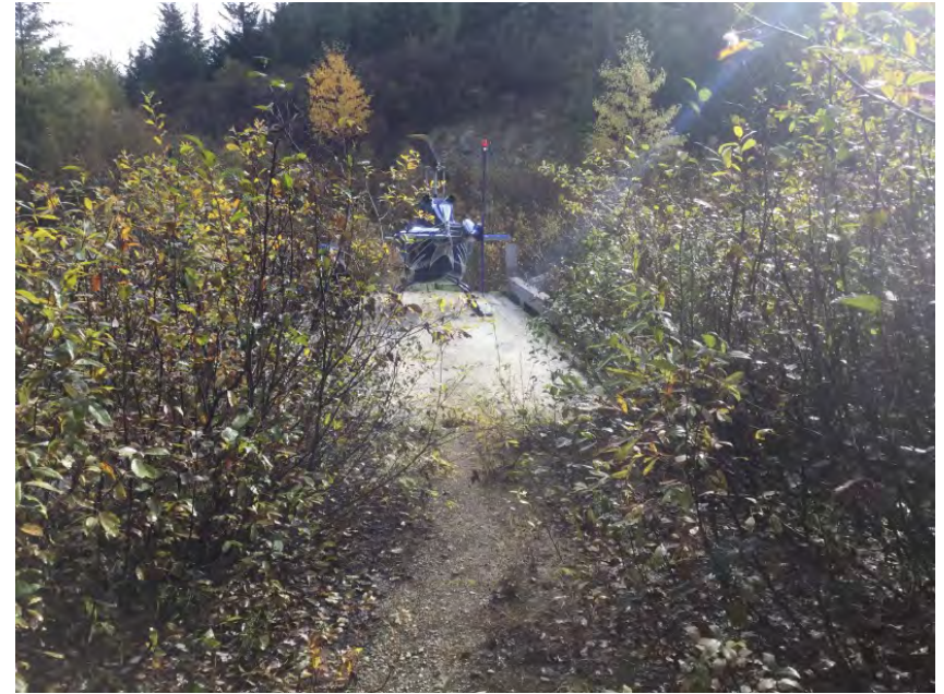
Approach from Left Bank when facing downstream
