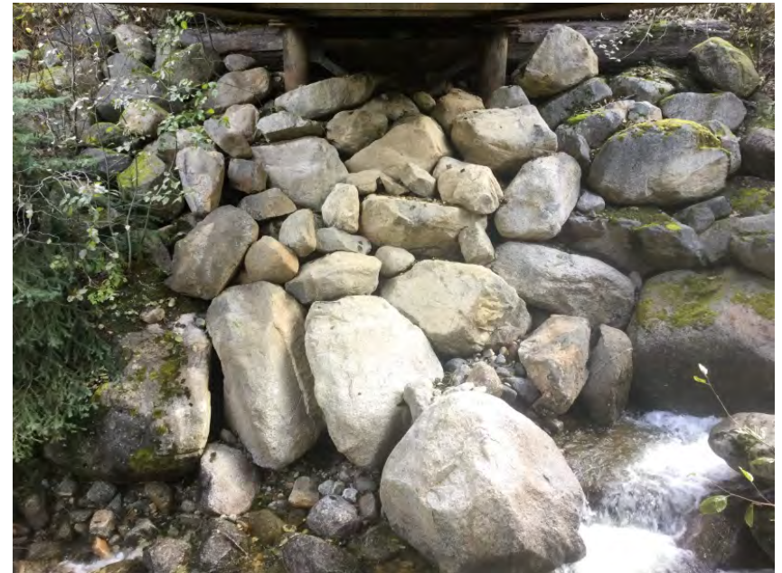
Right Bank Abutment when facing downstream
